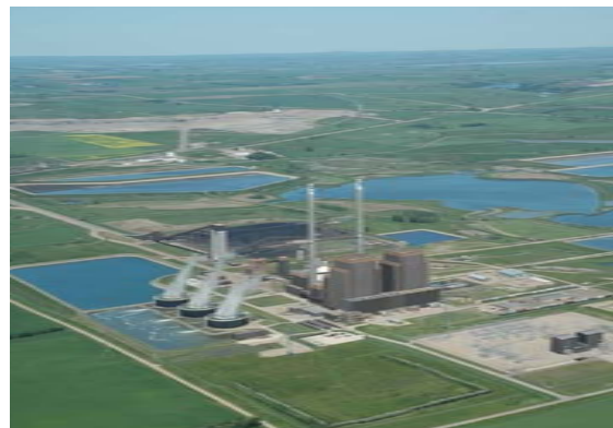
Great River Energy's Coal Creek Station - Underwood, North Dakota
